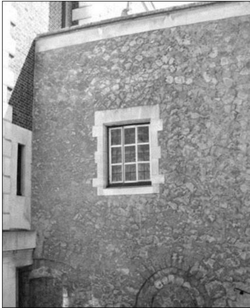
Fig. 44 The remaining part of the original Templar dining hall
